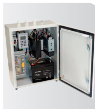
on industrial computer mounted in the RPD radio access unit
